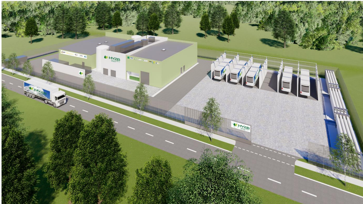
Green hydrogen electrolyzer from Hy2B Hydrogen GmbH with 6 filling stations for compressed gas trailers, funded by the Federal Ministry of Digital and Transport in the HyPerformer model region HyBayern
